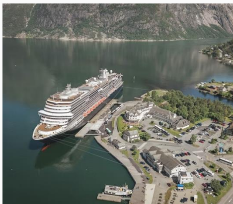
Eidfjord: Overview of the quay
